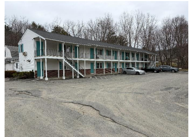
Figure 4- Secondary hotel Building to be demolished, looking east.
