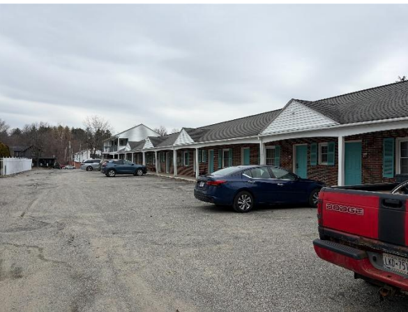
Figure 3- Primary hotel building to be demolished, looking west.
