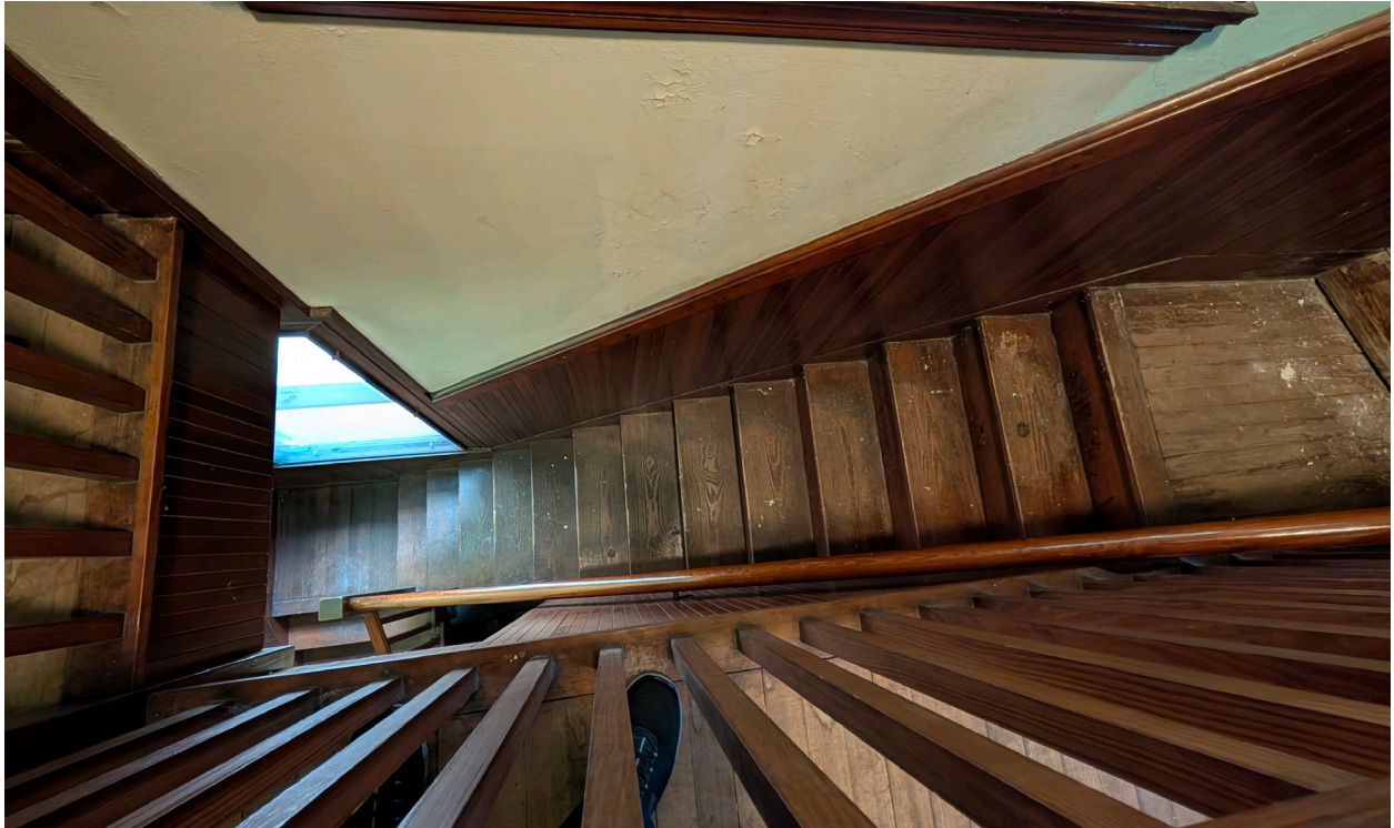
Narrow egress staircase
