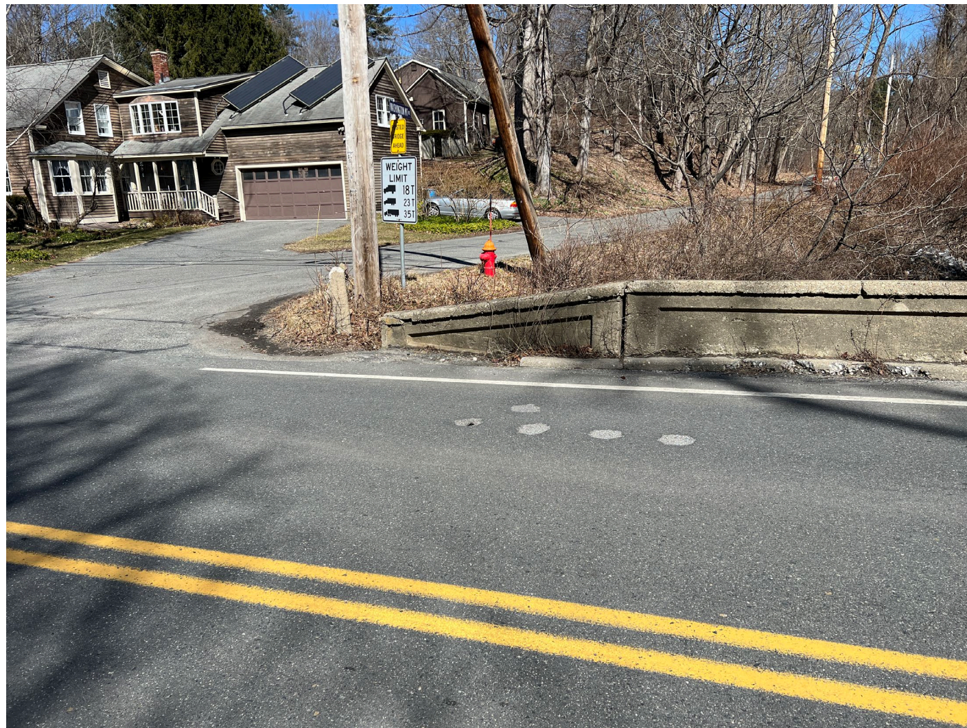
Lack of guardrail protection of railing.
