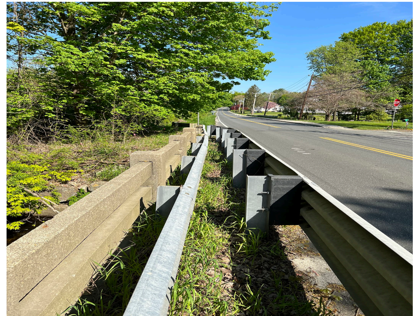
Poor condition of original concrete railing & steel beams below.
